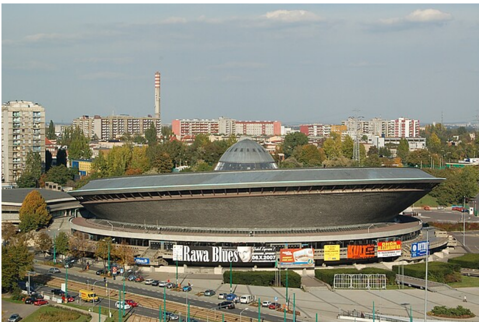
One of Katowice's main attractions, built in the Gierek-era: the UFO-style multipurpose arena complex hosting sports and cultural events
