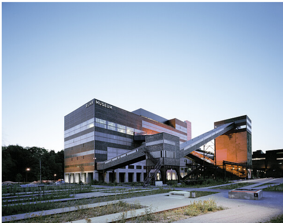
The former coal wash hosts the Ruhr Museum today Author: Brigida González, Source: Ruhr Museum
