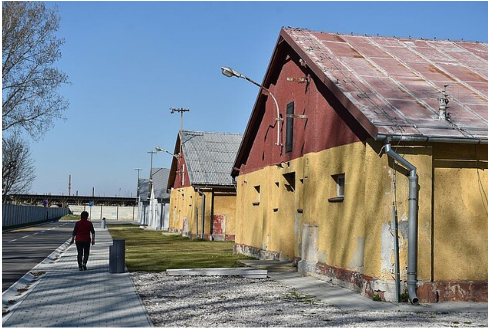
The barracks of the former Sered' camp
