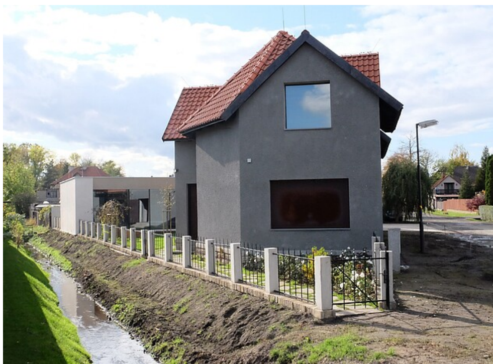
The Palach Memorial, all windows screened with metal plates Photo: Jakub Jareš
