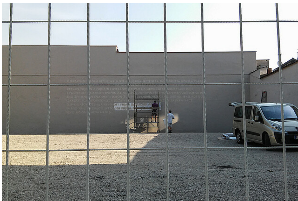
The construction of the Victims of all Wars Memorial, 6 July 2015
