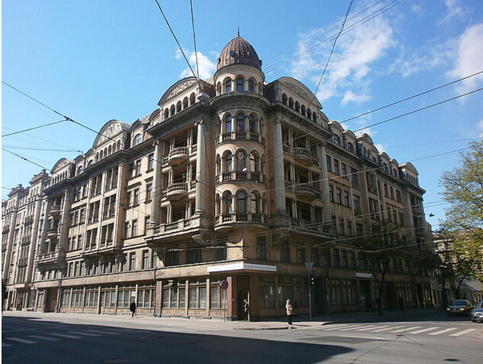
The former KGB headquarters on Brīvības street in Riga
